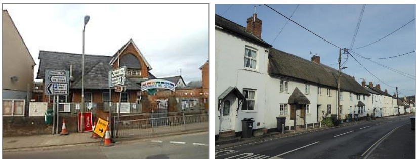
Examples of detracting features in Conservation Areas: Cluttered signage at Ottery St Mary (2013) and overhead power lines at Sidford (2018)
