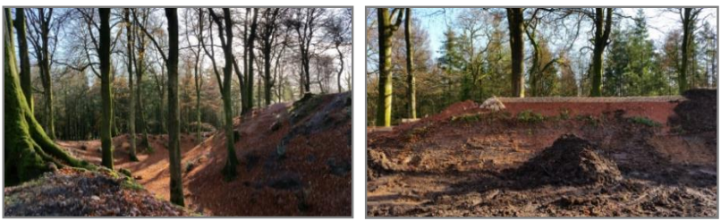
Woodbury Castle restoration project 2017- 2018, Woodbury Common.
